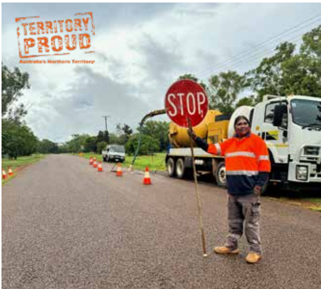
Sam on-site at an emergency job..
